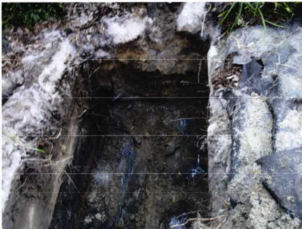
Picture 2: UST 754Althea excavation in progress.
